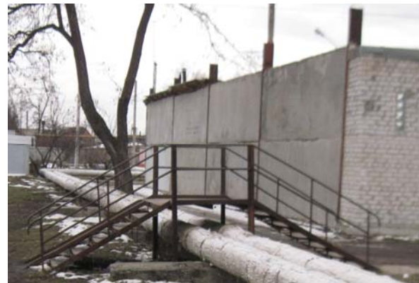
Figure 1. A bridge over the Kharkiv city pipeline.
